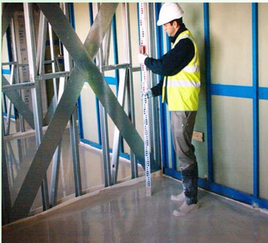
Checking the levels
