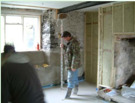
Checking the levels.
